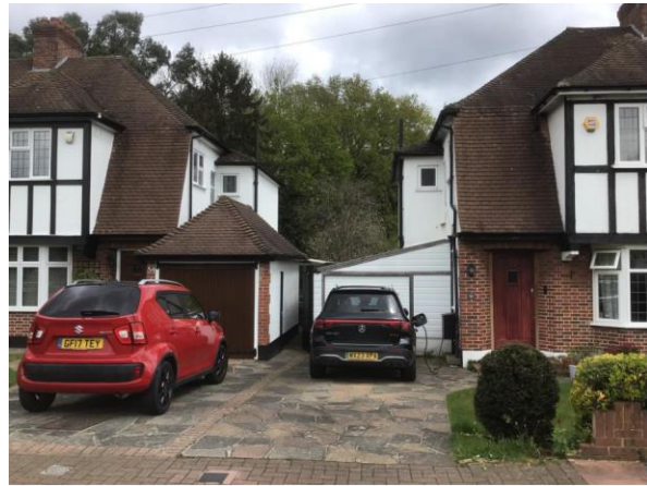
Figure 8: Nos. 54 (left hand side) and host dwelling (right hand side of image)
